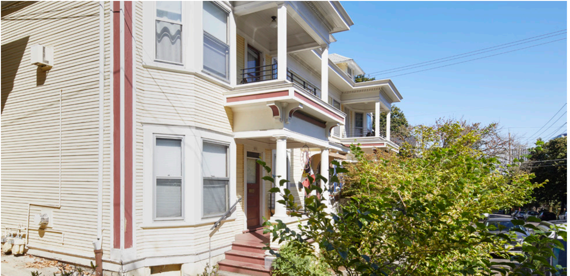
A historic South Portland plex exhibiting projecting bays.
