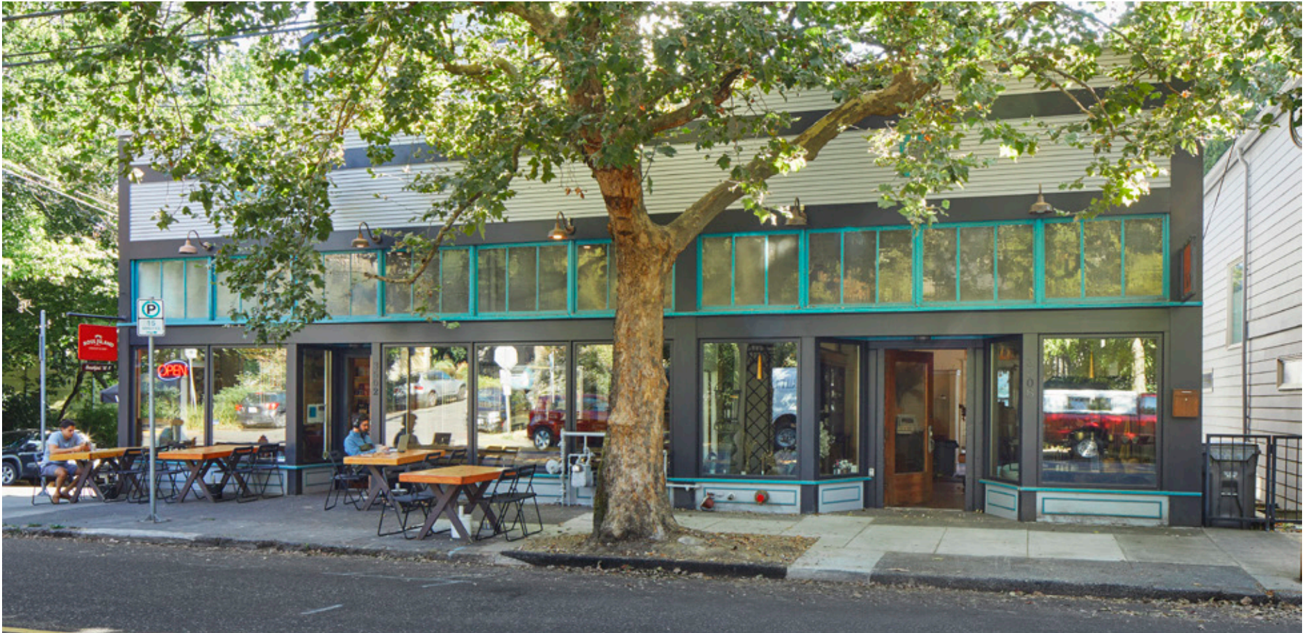
A mixed-use building in South Portland exhibiting entries typical of the typology.
