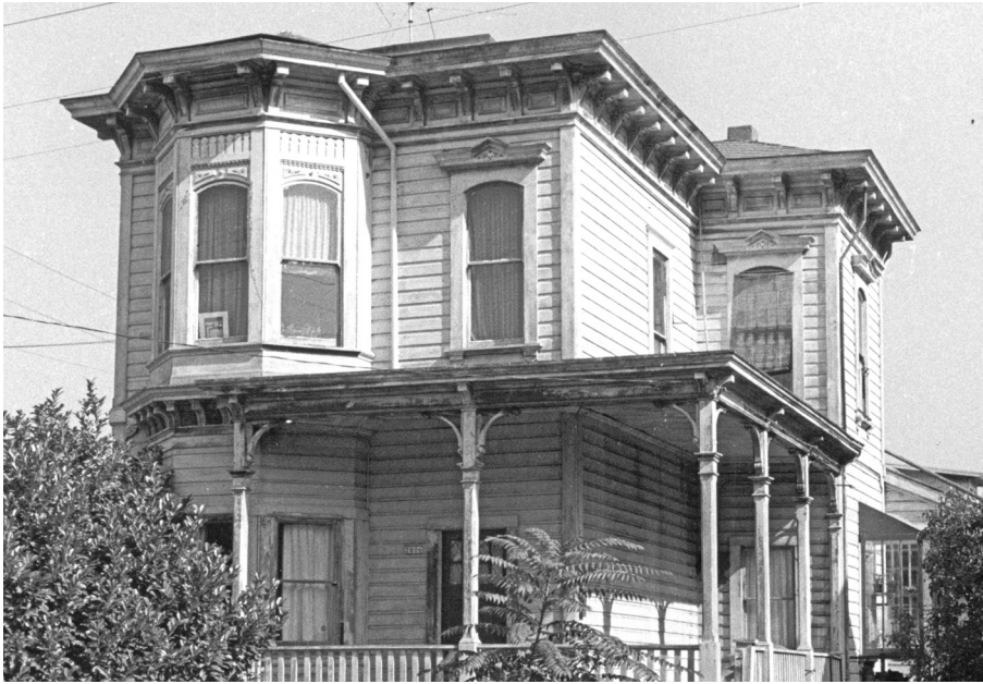
The Peter Taylor House exemplifies the Italianate style as found in South Portland. Image courtesy Norm Gholston.
