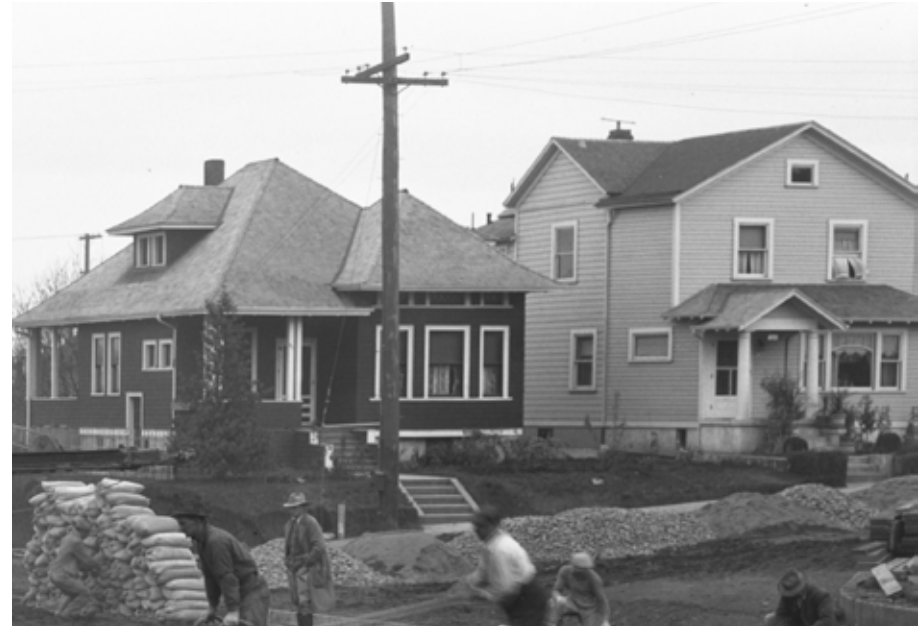
Although outside of the Historic District, this 1926 photo of the Ross Island Bridge under construction shows representative examples of the craftsman/bungalow styles found in South Portland. Image courtesy Portland City Archives, A2009-009.486.
