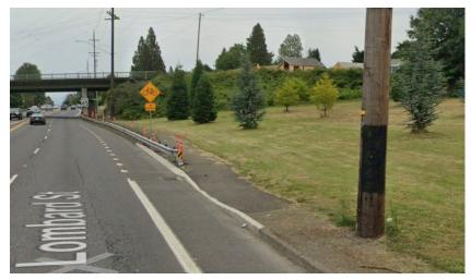
• WB direction: Approximately 500 linear feet of improvement along NE Lombard. Widen to 6' min bike lane and using 2-horizontal to 1-vertical slopes into the UPRR ROW. Outside travel lane may be narrowed to 11' to accommodate this widened shoulder in places as required. A design exception is anticipated for these roadway cross sections.
