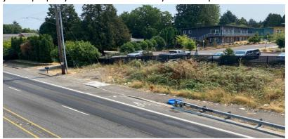
Begin new concrete sidewalk on west end with ODOT ramp details, matching to existing MUP access point shown below. This allows for future ODOT projects to connect to a new sidewalk.
