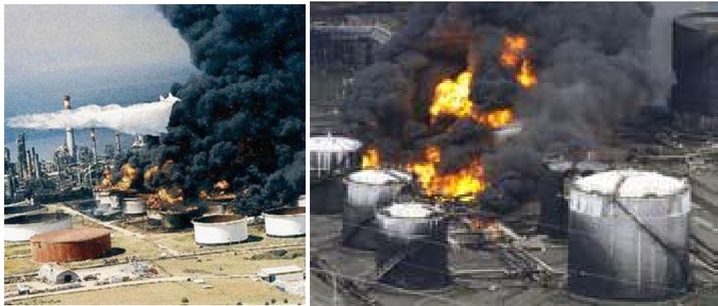
Figure 5: Fire Caused by Tank Damage following 1999 Turkey (left) and 2011 Tohoku Earthquakes (right) (French Ministry of Ecology, Sustainable Development and Energy, 2013)
