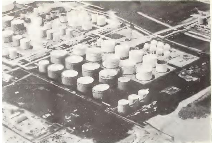
Figure 3: Spilled Oil Past the Containment Dikes following 1978 Earthquake in Japan (NBS 1980)
