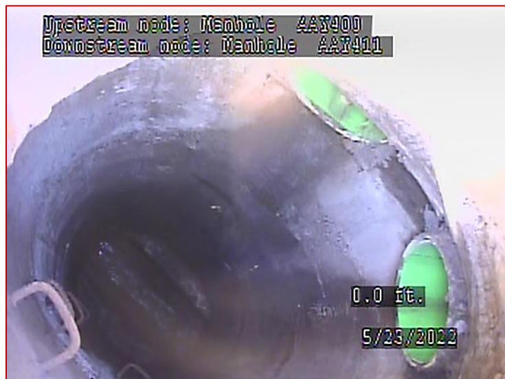
Photo 5: CCTV inspection photo of AAY400 on NE 33 rd Ave
