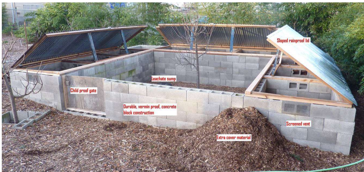
Figure 4. The compost processor with bin lids that also serve as a roof propped open for inspection and servicing. Notice the gate, screened vents, and pile of extra cover material at the front. A faucet with hose and sprayer is convenient for cleaning each batch of containers.
