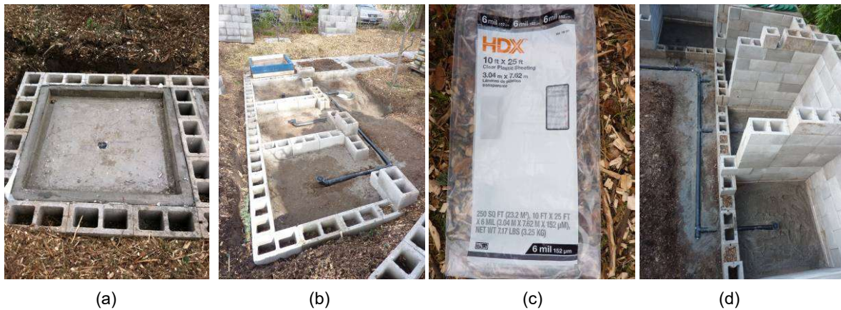
Figure 12. The bottom of each bin consists of a 4" thick, 48"x48" waterproof concrete pad sloped toward a drain in the center (a). The edge of this pad has a 4" tall lip to channel all leachate to the center drain (b). This photo shows the drain plumbing prior to placement of the vapor barrier and pouring the concrete pad (c). A 6mil vapor barrier was placed under each concrete pad (d). The drain outside Bin 1 has a cleanout.
