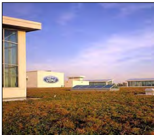
American Honda in Gresham incorporates a highly reflective roof, rainwater harvesting and passive air conditioning systems.
