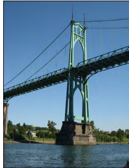
The majestic St. Johns Bridge soars above the North Reach of the Willamette River.
