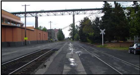
Rails in roadway along N Bradford Street.
