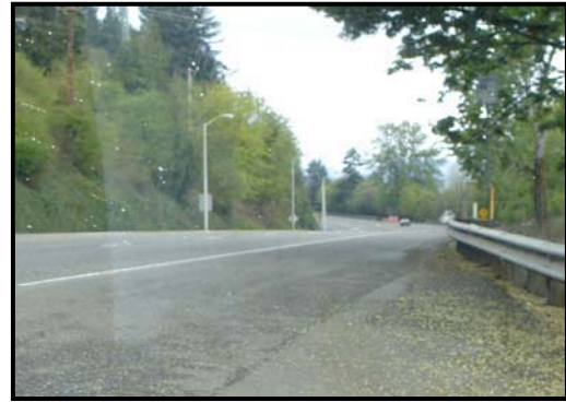
Potential sight distance issue looking north on US 30 from NW Marina Way.
