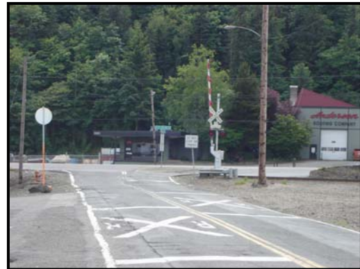
Right turn channelization and railroad crossings at NW Balboa and US 30.
