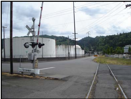
Rail crossing in intersection at NW 61 st Ave and NW Front Ave.
