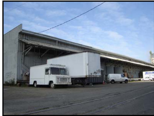
Poor pavement conditions on N River Street in front of site.
