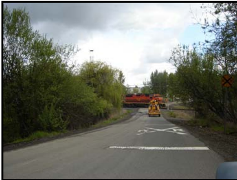
At-grade rail crossing on NW Marina Way.
