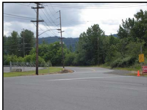
Sight distance issue at intersection of N Time Oil Rd and N Burgard St.
