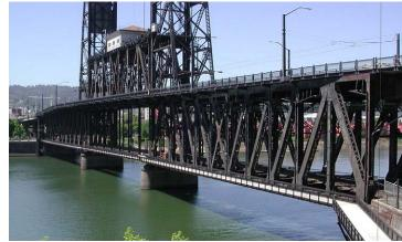
The Steel Bridge in Portland, combination rail-roadway-light rail lift bridge carries a multi-use trail adjacent to the lower lift deck.
