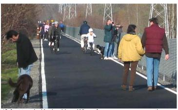
12-foot tread with shoulders. Where fences are necessary, they should be at least 12" from edge of tread (Springwater-OMSI Trail).
