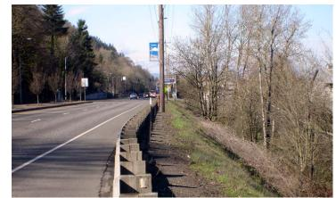
The existing ground falls away steeply. Some places include retaining walls very close to the guardrail and industrial facilities adjacent to the right-of-way.
