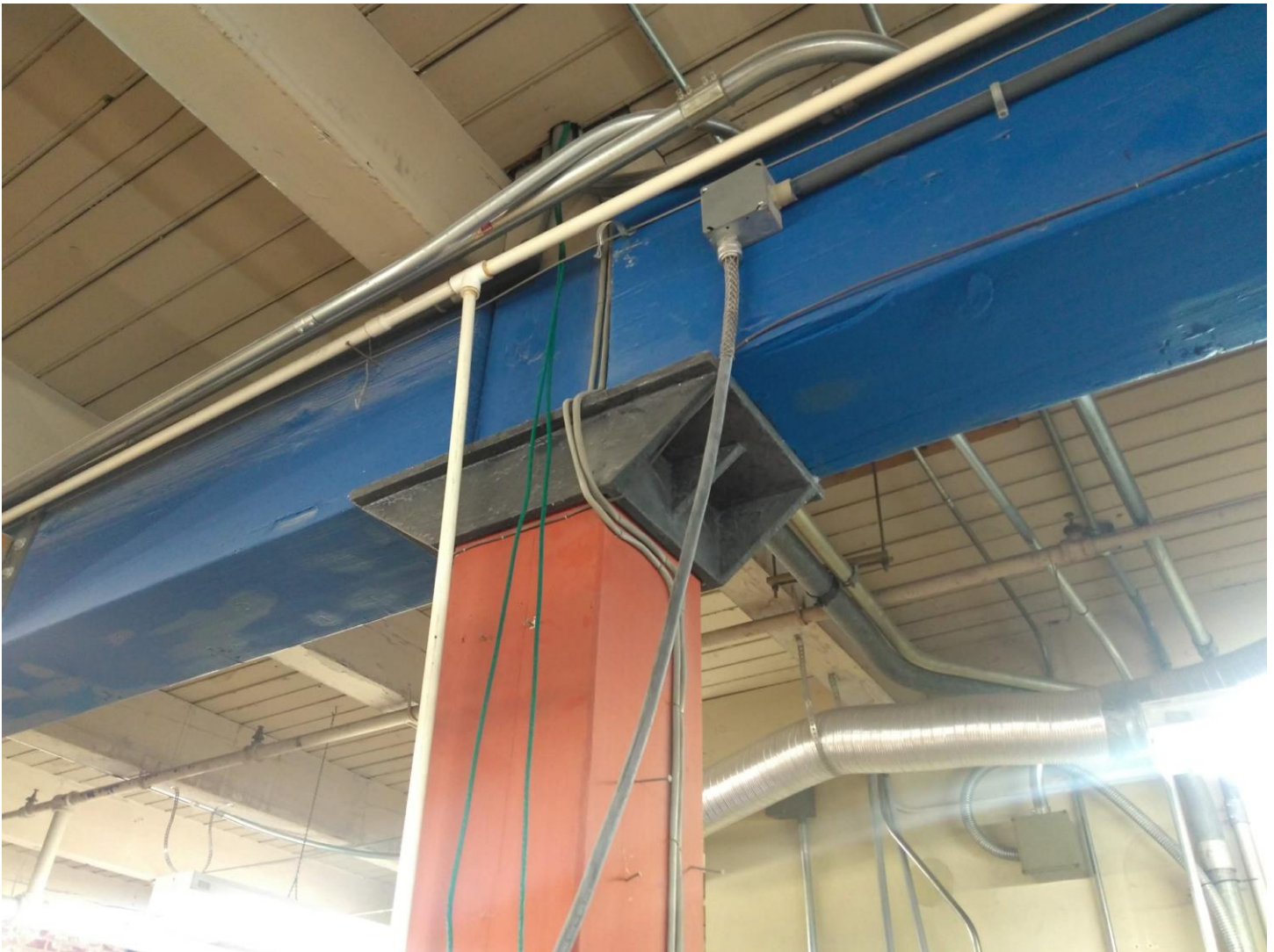
Figure 1: Existing condition between the 2-hour column and 2-hour beam assemblies
