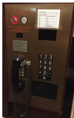
Figure 19 - Elevator recall at FCC (Panel 2)
