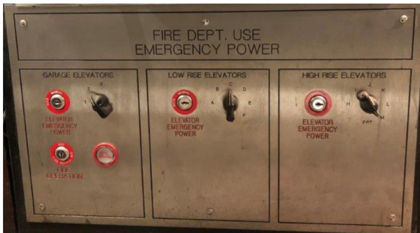
Figure 20- Elevator Emergency Power Selection Switch
