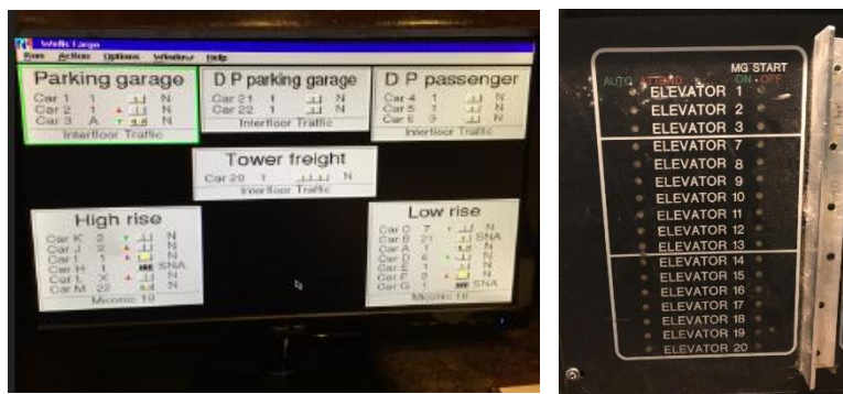
Figure 8 - Elevator Location and Operation Status Panel and non-functional legacy panel.
