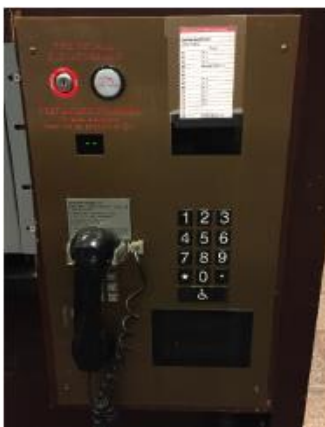
Figure 18 Elevator Recall Panel at FCC (Panel 1)
