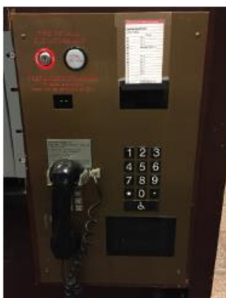
Figure 18 Elevator Recall Panel at FCC (Panel 1)
