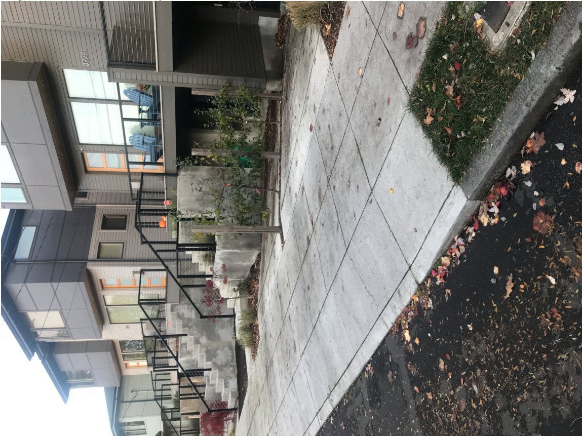
Driveways and sidewalks to be demolished to allow for new/additional connection. Existing 3" runs diagonal across both driveways before entering the street.
