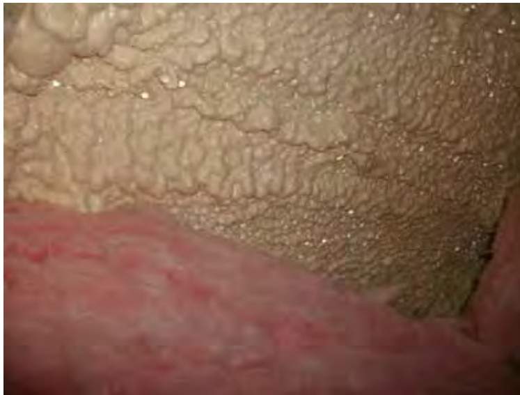
Figure 3. ccSPF unvented roof with condensation
