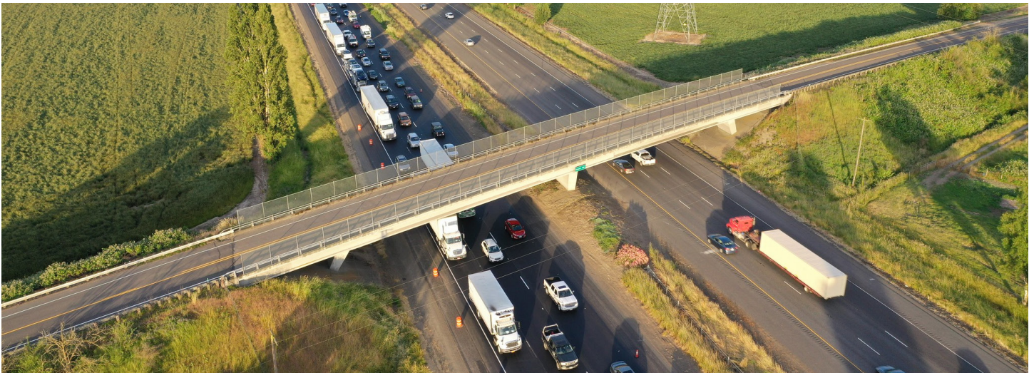
Picture 5.1: Aerial image of a divided freeway under an overhead bridge. Multiple white freight trucks and passenger vehicles of varying sizes and colors are driving through the freeway. [Source: ODOT]
