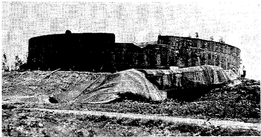
*Figure 1: Failed Tank following 1933 Long Beach Earthquake (Cooper 1997)*
