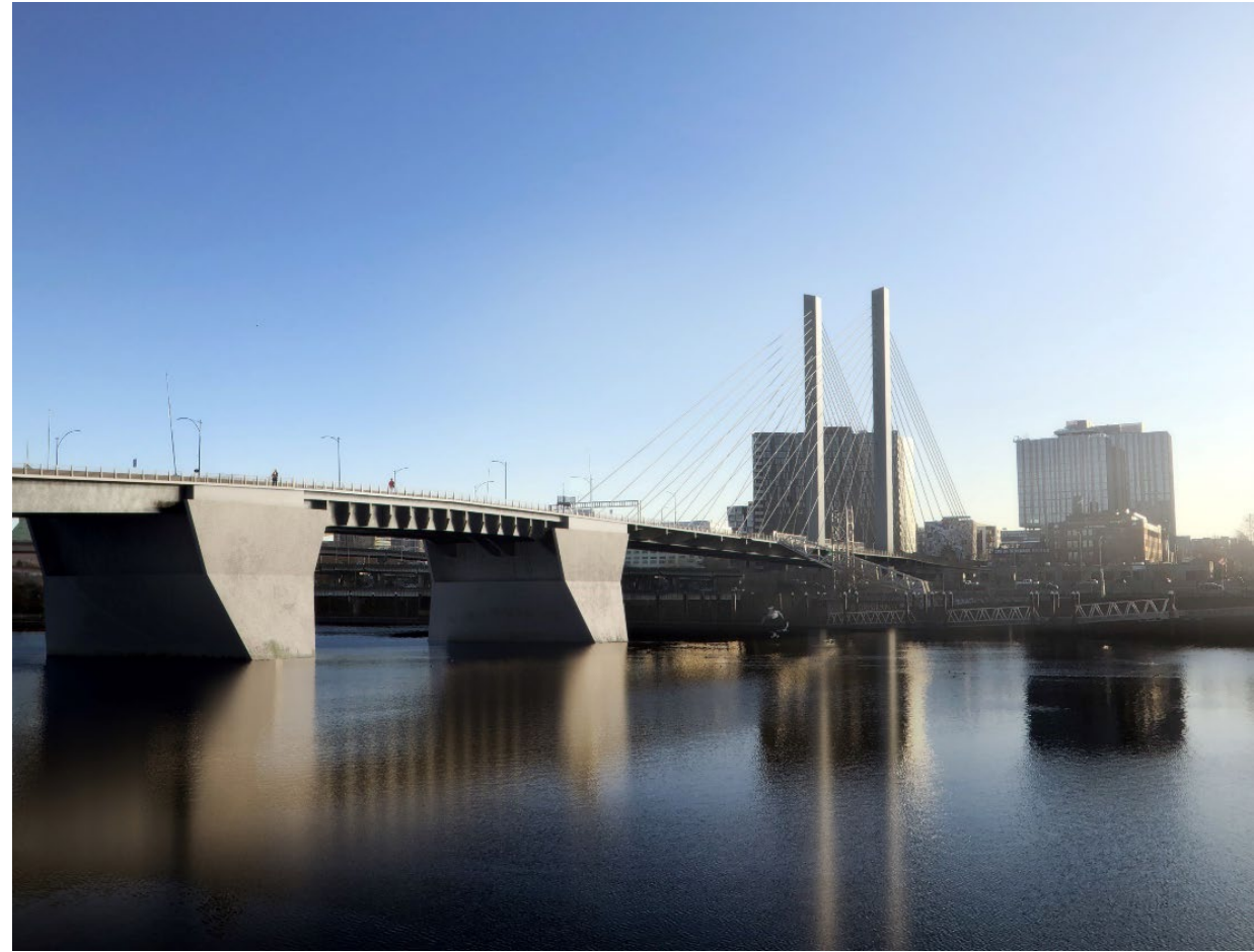
Replacement Long Span with Cable Supported
