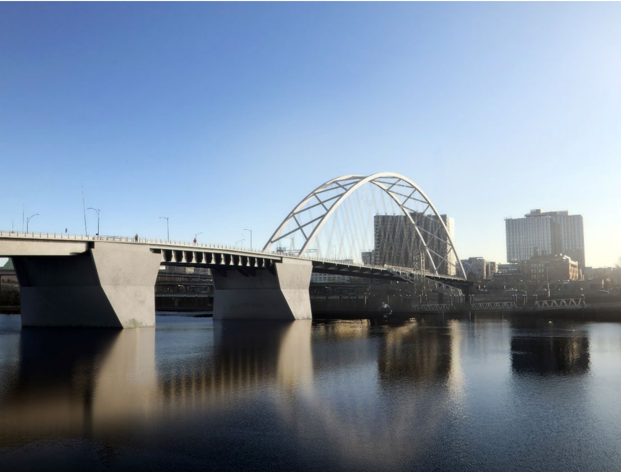
Replacement Long Span with Tied Arch
