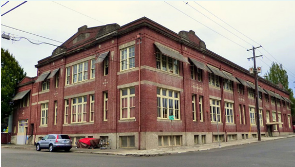
Troy Laundry Building, URM, currently under renovation including seismic retrofit
