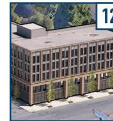
12 STARK ST FAMILY HOUSING New Construction
