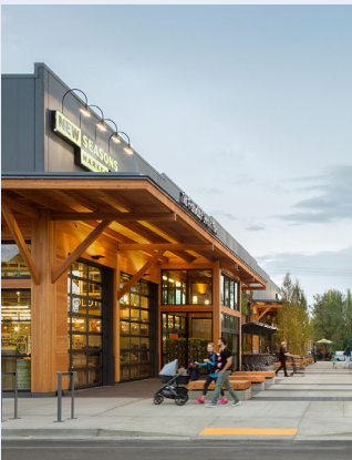
Commercial storefront utilizes a set-back frontage to extend the public realm, providing hardscaped areas, seating and large operable doors.
