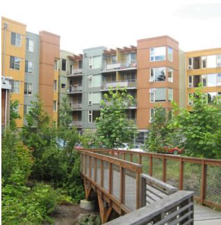
Multnomah Village uncovered and restored Tryon Creek headwaters, supporting natural habitat and functions.
