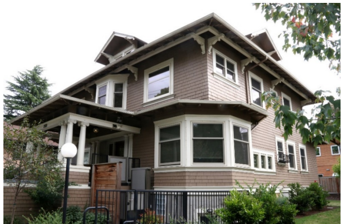
Use flexibility allowed this former single-family home in SE Portland to evade a proposed demolition and be repurposed into seven rental homes.
