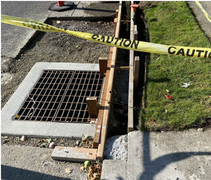
Inlet Installation
