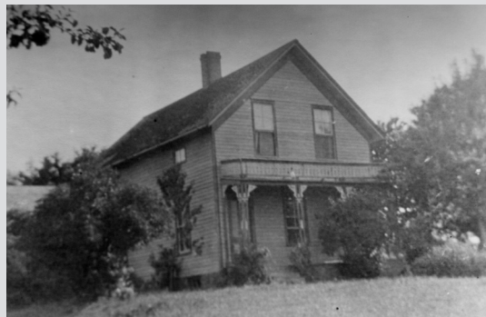
Historic image of the Carman House, Lake Oswego, OR.
