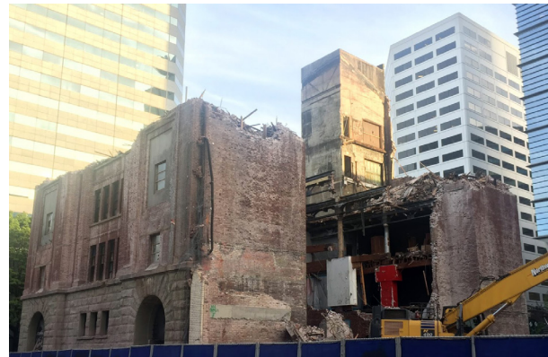
Demolition of the United Workmen Temple, September 2017
