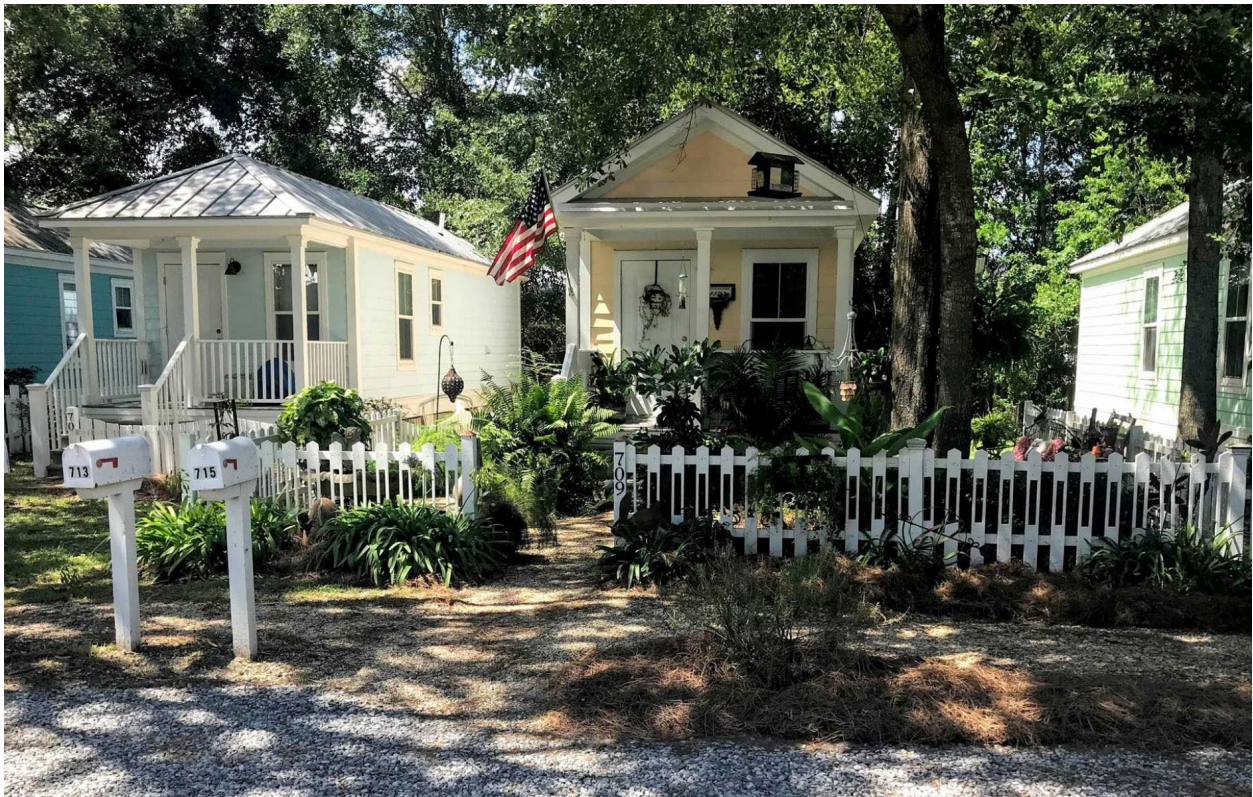
Mississippi Cottages, Ocean Springs - built 2008
