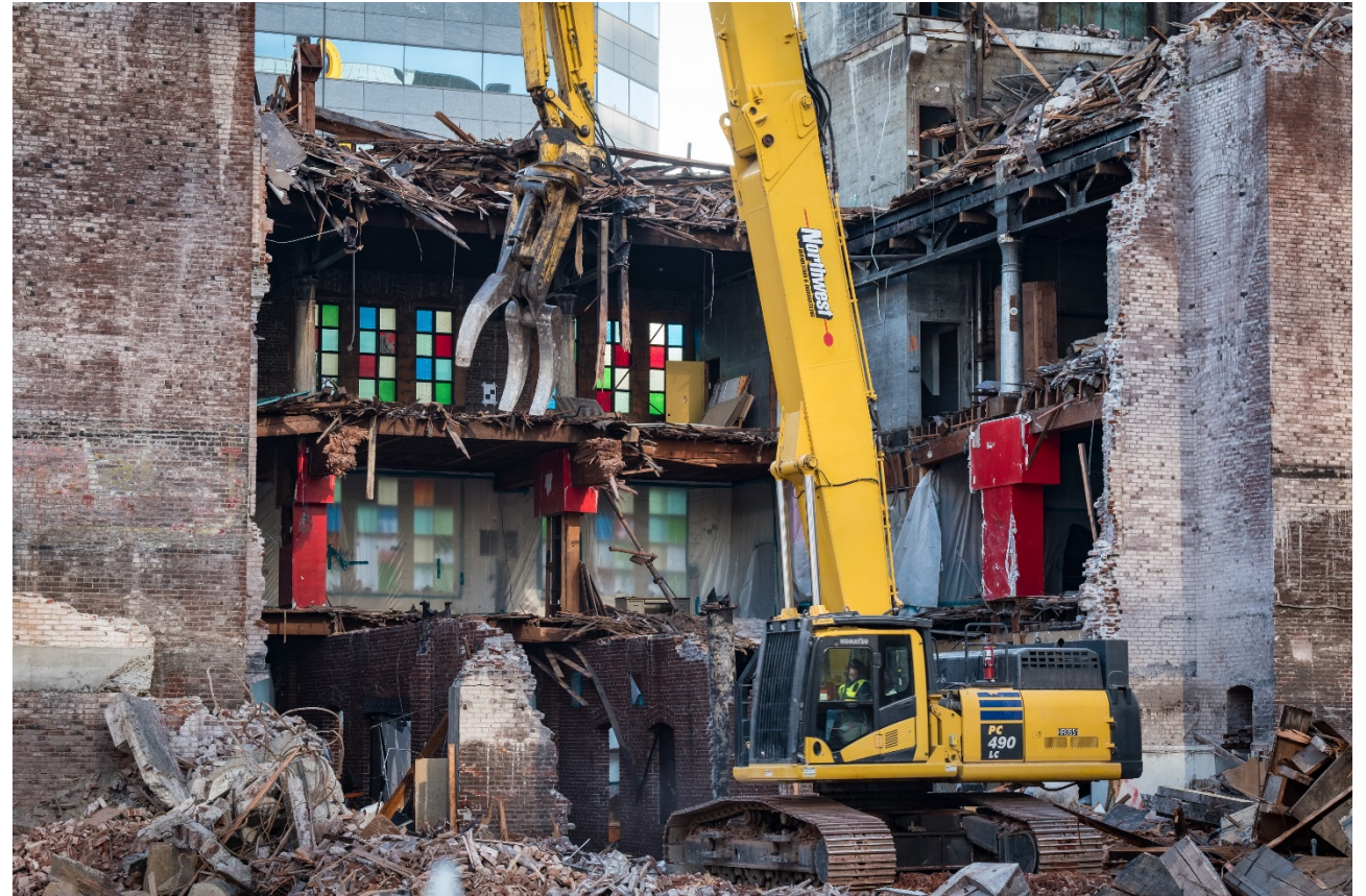
Demolition of a Significant Resource. Photo: Scott Tice.
