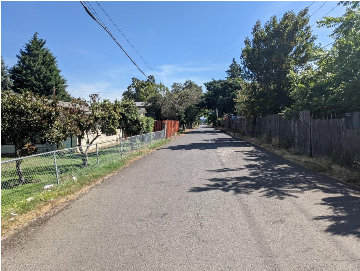
This road in the project area is paved, but there is no sidewalk or pedestrian protections
