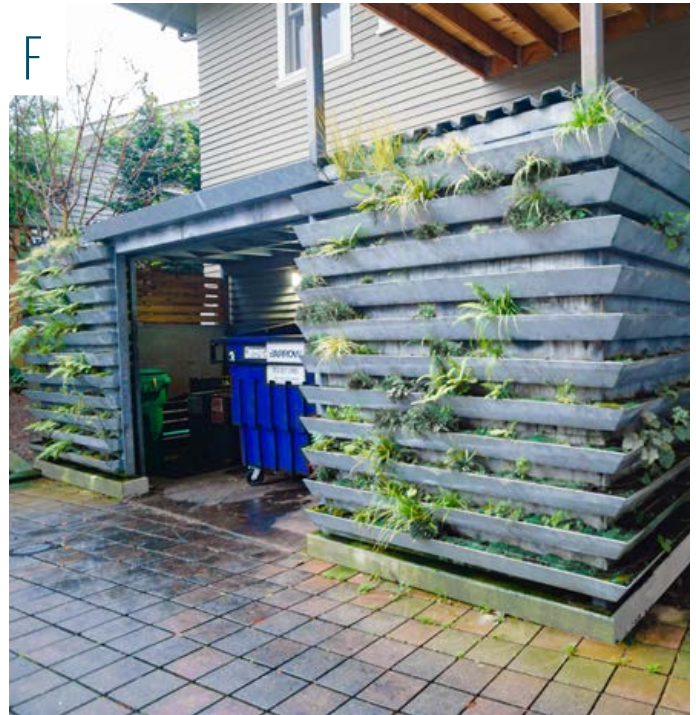
Tucking and screening waste bins. This trash and recycling area is well-hidden from the building's street-facing façade and artfully screened behind a planter designed to capture rainwater. Division, SE Division and SE 38th
