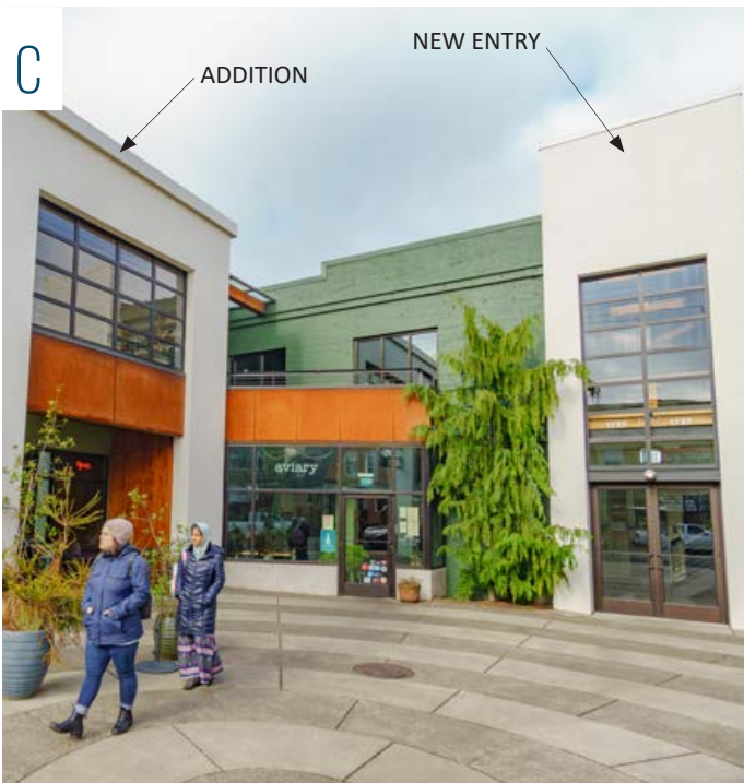
Creating an addition that references existing architecture. This addition integrates similar materials in its new entry and the new building and connects both with special paving and a shared courtyard. Alberta, NE Alberta and NE 18th
