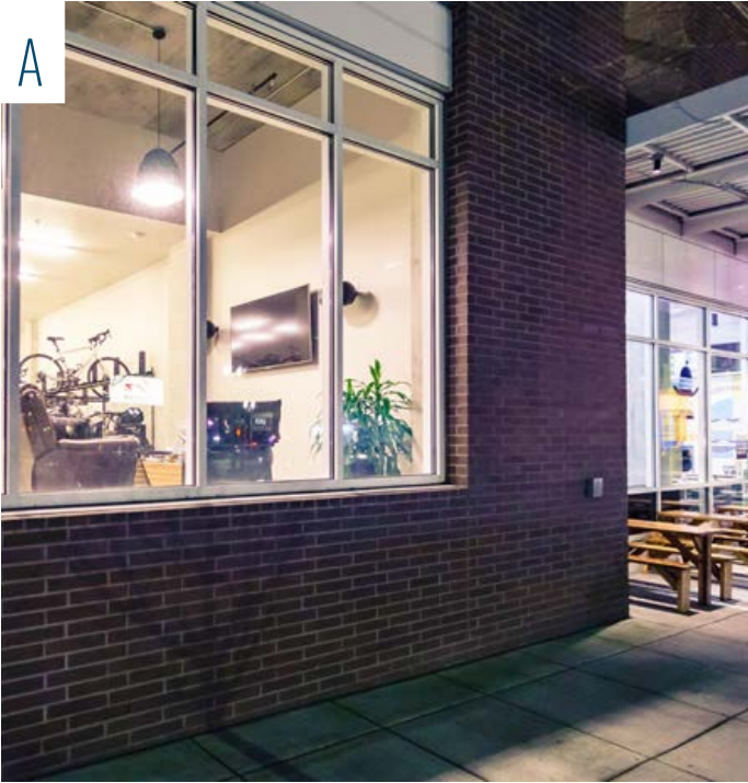
Activating bicycle parking along the building's ground floor with windows that face an interior lobby and bike repair amenities. Central Eastside, SE Morrison and SE 6th
