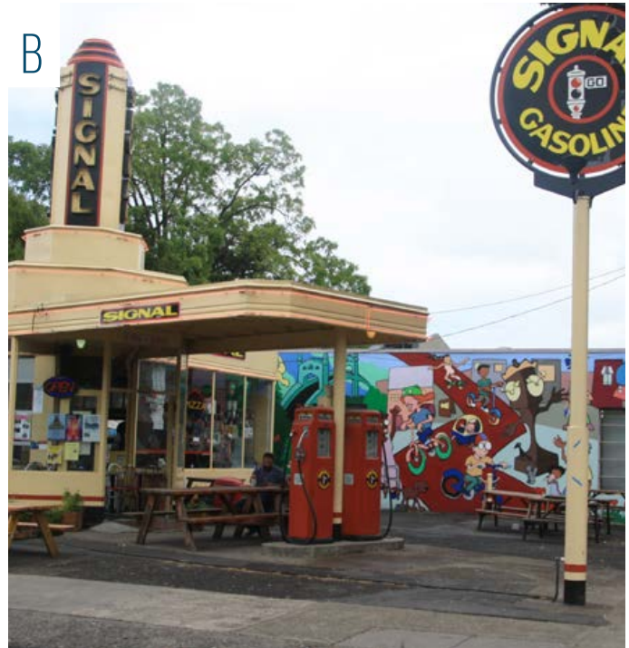
Maintaining a site's uniqueness by re-purposing architectural elements, such as sculptural neon signage and character defining canopies. St. Johns, N Lombard and N Charleston
