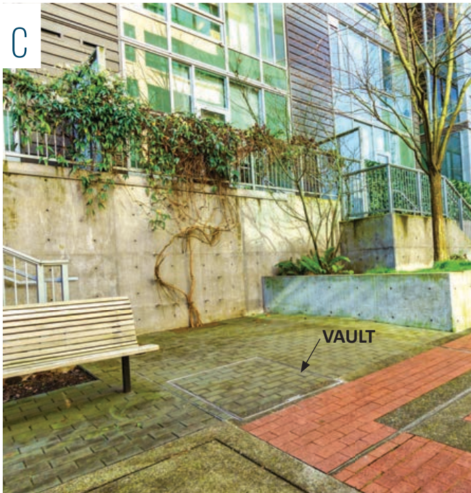
Integrating vaults into the paving design. This underground utility is well-hidden, while the design of the space includes room for trees. South Downtown/University, SW Mill and SW 4th
