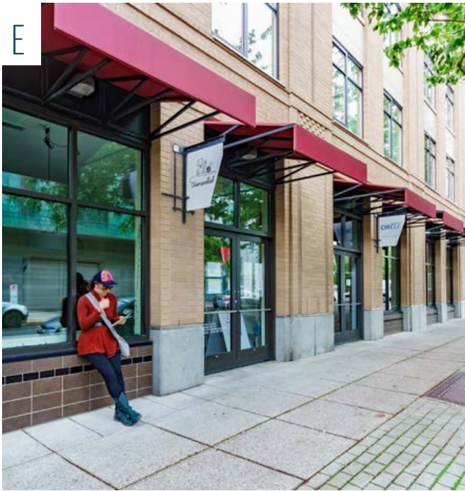
Shaping seating opportunities on fully built-out sites. Designing wide sills or leaning rails as seating can have large impacts on expanding the public realm. Pearl, NW Overton and NW 11th Ave
