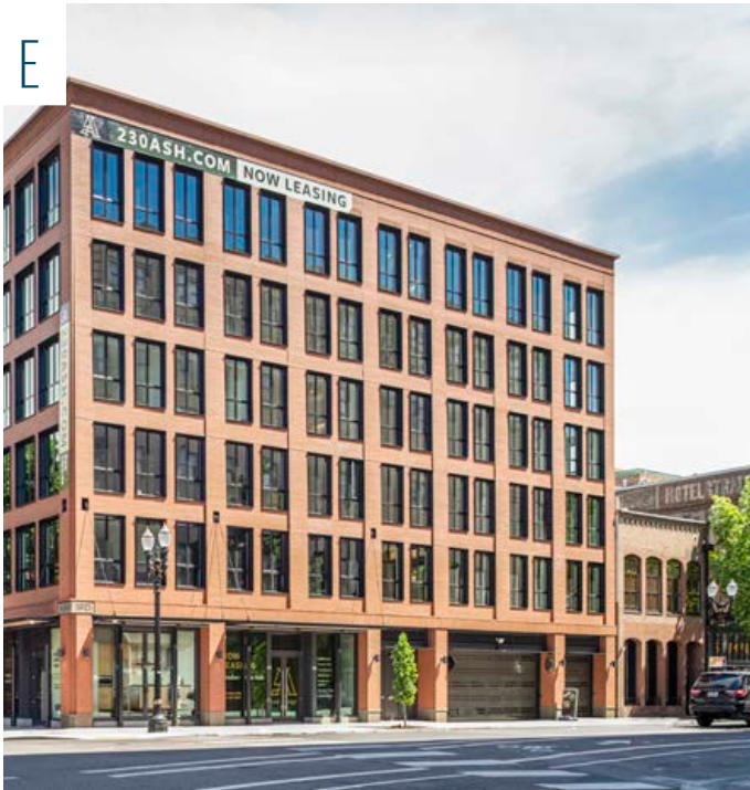
Aligning belt courses and window heights. This newer building on the left uses the same vocabulary as its historic neighbor: materials, repetition of bays and windows, and continuity of setbacks. Old Town/Chinatown, SW 3rd and SW Ash
