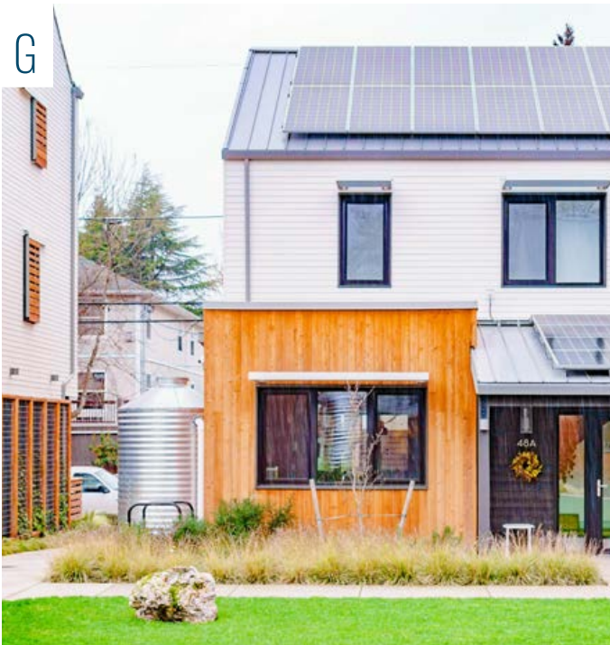
G Striving towards net zero with features that include photovoltaic panels on all south-facing roofs, triple-paned windows to limit the amount of hot and cold air and cisterns for collecting rainwater. Eliot, NE Williams and NE Tillamook
