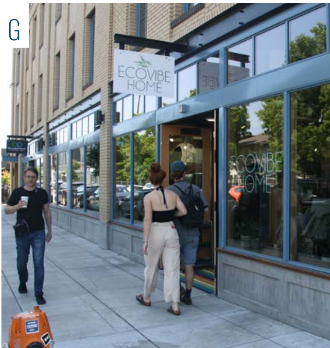
Drawing on traditional materials and patterning to create an organized and articulated ground floor. Heavy masonry materials, such as brick and concrete extend to the ground to express the building's structure. Alberta, NE Alberta and NE 19th
