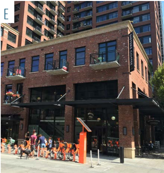
E Reusing salvaged brick in the façade of new buildings. This example references its site's history and conserving valuable resources. Pearl, NW Marshall and NW 13th
