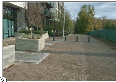
2 ENRICHED PAVEMENT AND FORM LINED PLANTERS
