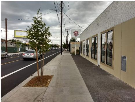
**Foster Streetscape Project:** East of SE 82<sup>nd</sup> Avenue the project provided wider sidewalks, bike lanes, street lighting, and new paving, by means of a four-to-three lane road reorg and moving the curbs inward. The combined federal aid and Fixing Our Streets project was completed in 2019 and extends from SE 52<sup>nd</sup> Avenue to SE 90<sup>th</sup> Avenue.
