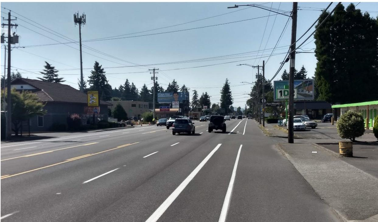
Figure 17 - NE Halsey Street, looking west from NE 118th Avenue. Little-used on-street parking would be repurposed for protected bike lanes with concrete separators.
