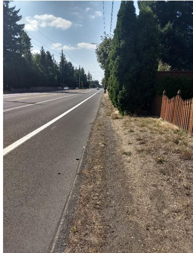
Figure 3 - Missing sidewalk on NE Halsey Street.
