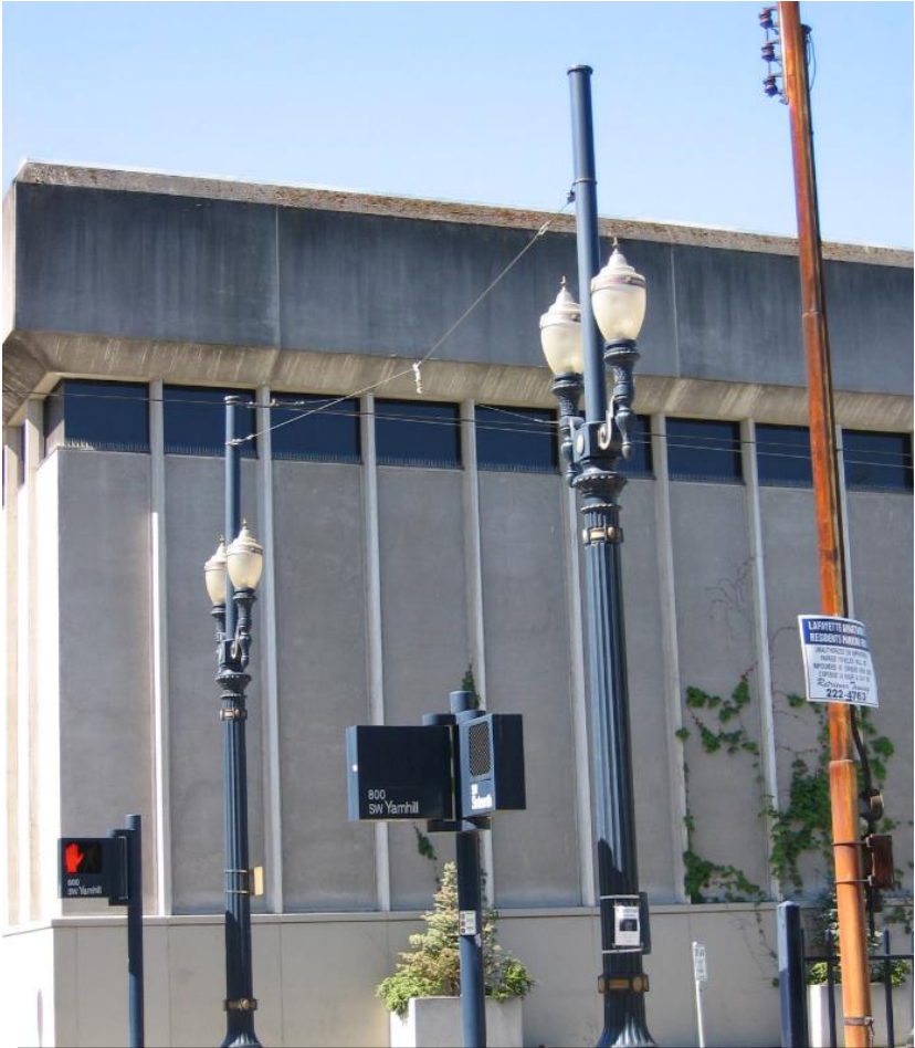
Concept for dual use pole began in 1986 with Banfield Light Rail Downtown. The Twin Ornamental was re-engineered to accommodate a full-height steel pole within the outer ornamental cladding.
