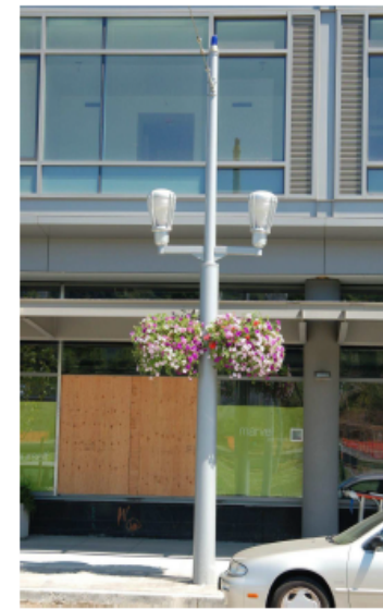
South Waterfront street light is an example of a twin luminaire fixture with clean attachment of support arms and an energy-efficient luminaire.
