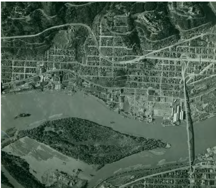
1950 Aerial Photo in South Reach
