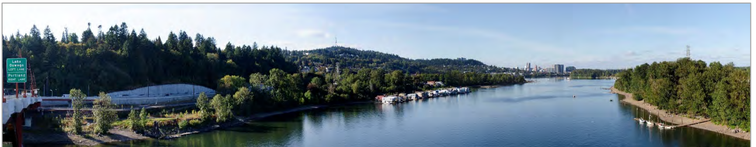
View from north side of the Sellwood Bridge with the Willamette River and the downtown skyline in the distance.
