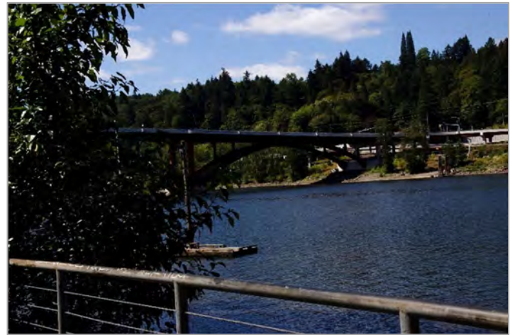
View of Sellwood Bridge with vegetation obscuring view.
