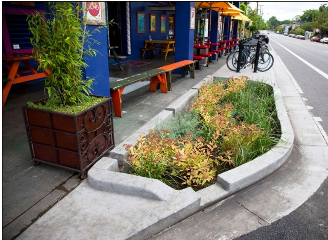
Curb extensions are street-side landscape areas that store, filter, and often infiltrate stormwater runoff. The curb extension shown above does not use the furnishing zone. Photo credit: Henry Ngan.
