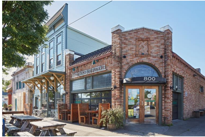
Historic resources in the Woodlawn Conservation District.
