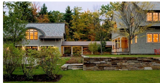
Connected accessory structure
