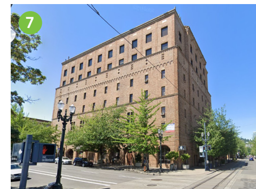
Brick bldg across 405
