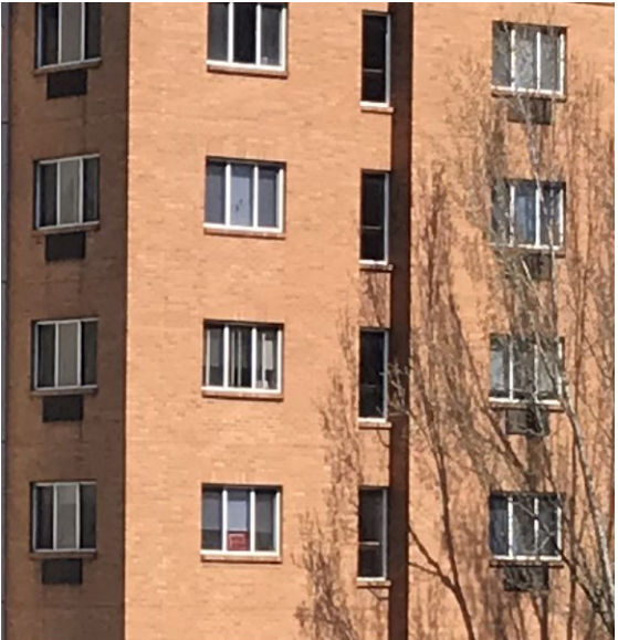
MATERIAL: EXISTING BRICK
