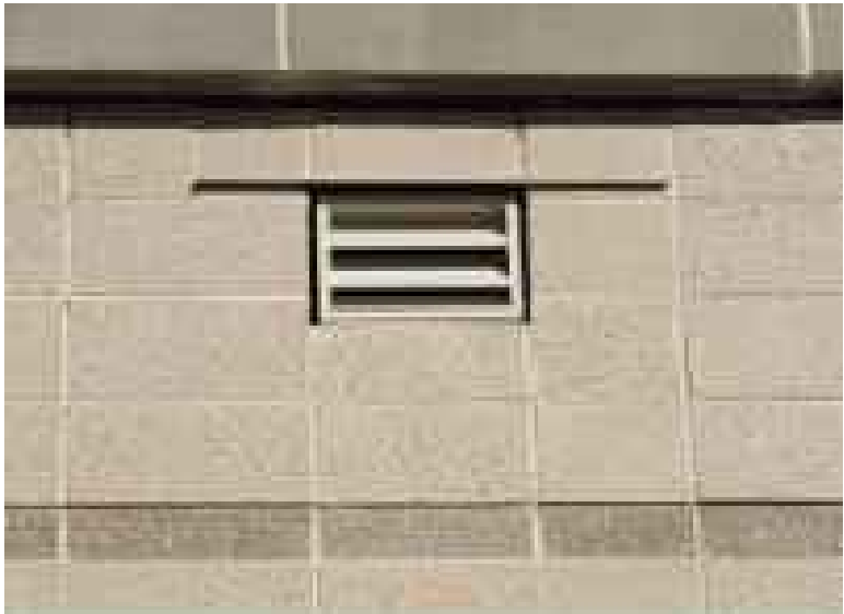
VENTING HIGH PERFORMANCE FIXED ARCHITECTURAL LOUVER FRAME: .060" EXTRUDED ALUMINUM (16 GA) COLOR: MATCH ADJACENT EXTERIOR CLADDING COLOR BRAND: UNITED ENERTECH
