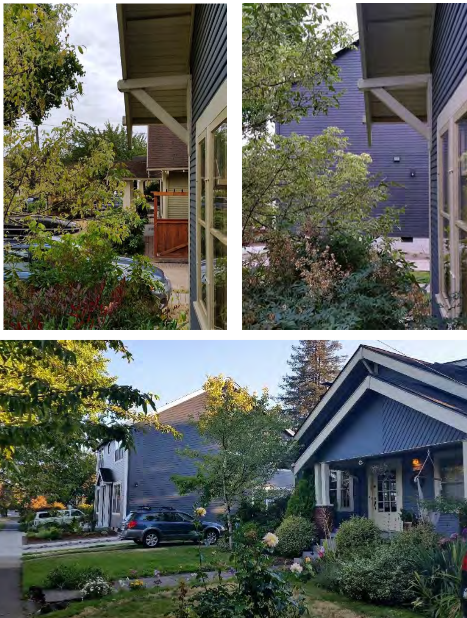
Figure 1: Visual effect of replacement of an existing home with a 32-foot setback matching adjacent homes (top left) by new construction with a 15-foot setback allowable under Proposal 3 (top right), and as seen from sidewalk (bottom). House shown at 3215 NE 42 nd Avenue.
