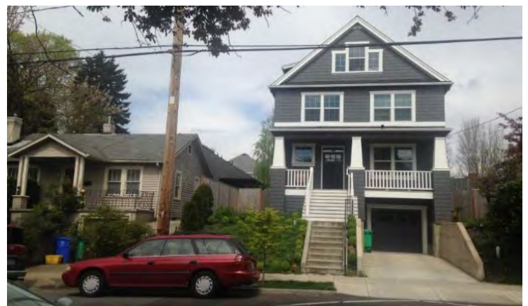
Narrow eaves, common in many new Portland houses, are often the result of current setback limits.
