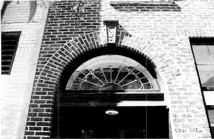
The Union Gospel Mission Building brickwork has highly contrasting mortar joints.
