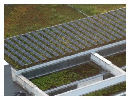
Figure 2. PV panels on large ecoroof in Basel, Swiss. 2013
