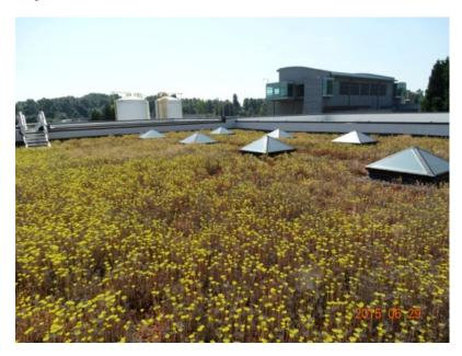
Figure 8 BES simple ecoroof at the Columbia Blvd. Wastewater Treatment Plant. It has no irrigation and the cost was \$6 sf in 2011 when it was installed.
