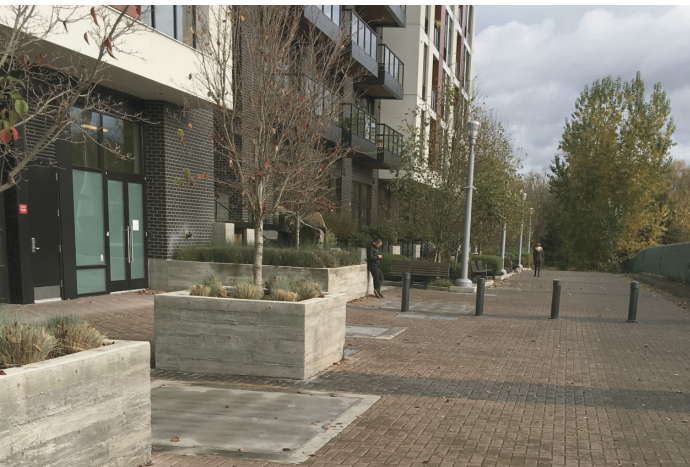
FORM LINED CONCRETE PLANTER ⑪
