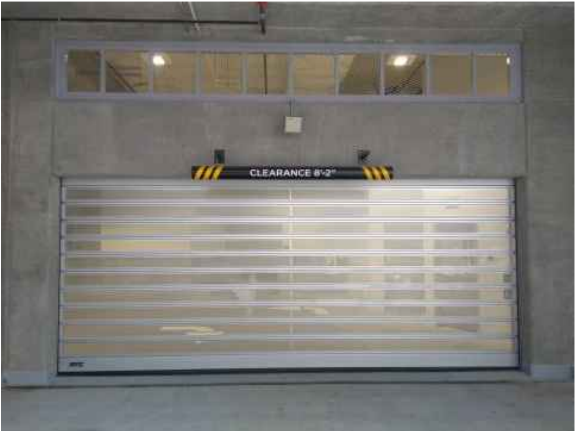
GARAGE DOOR SPIRAL VT - HIGH PERFORMANCE VENTILATED DOOR COLOR: RYTEC SILVER SIZE: WIDTH 20', HEIGHT 11' BRAND: RYTEC DOORS
