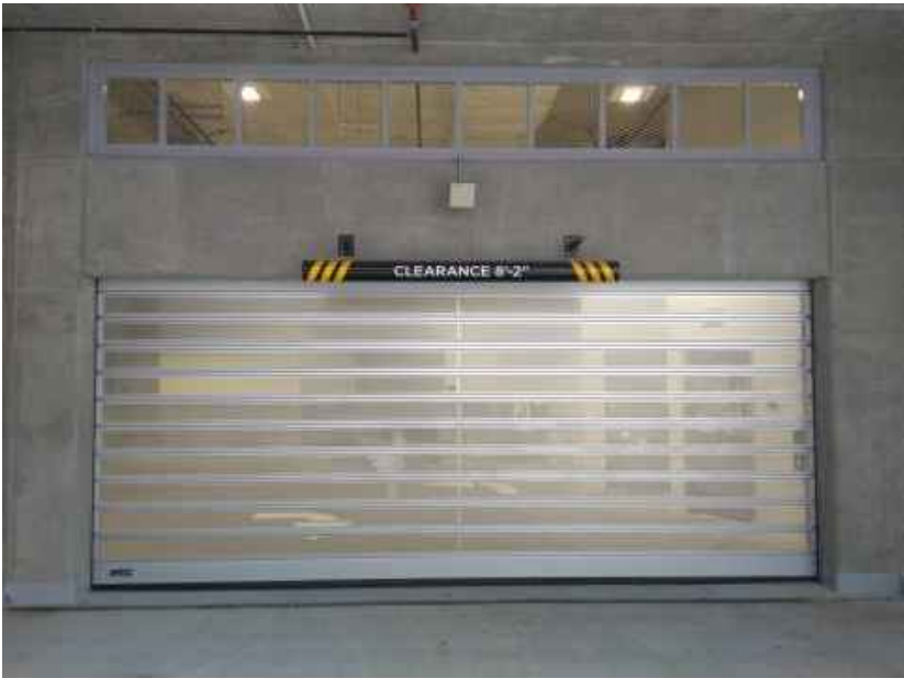
GARAGE DOOR SPIRAL VT - HIGH PERFORMANCE VENTILATED DOOR COLOR: BLACK SIZE: WIDTH 20', HEIGHT 11' BRAND: RYTEC DOORS
