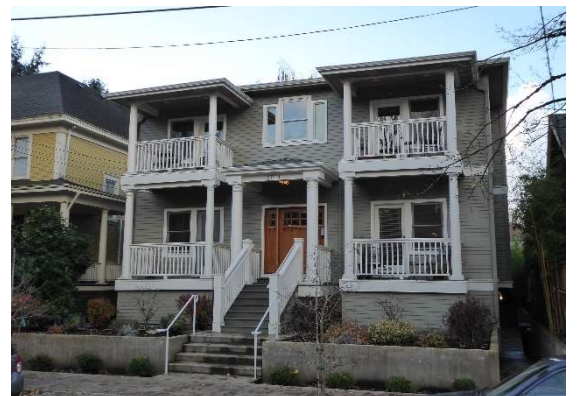
Recent five-plex project with no off-street parking, allowing it to fit into the neighborhood context.
