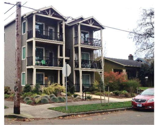
Landscaped front setbacks can help continue established neighborhood patterns, even with higher-density developments.
