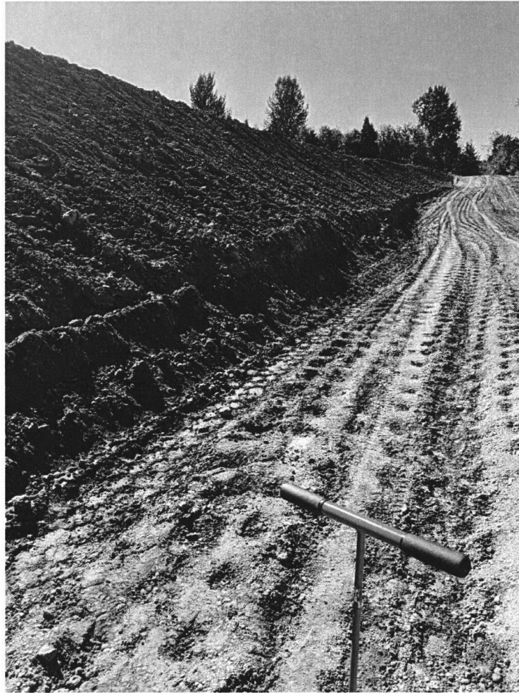
Photo 1. Strip of treated native subgrade on the West edge of the building pad, taken looking south
