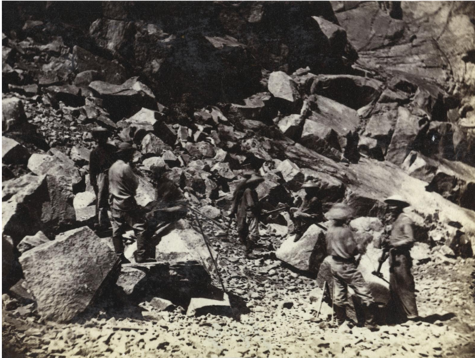
Chinese workers near an opening of the Summit Tunnel of the Central Pacific Road (1862-69), Hart, Stanford Univ.
