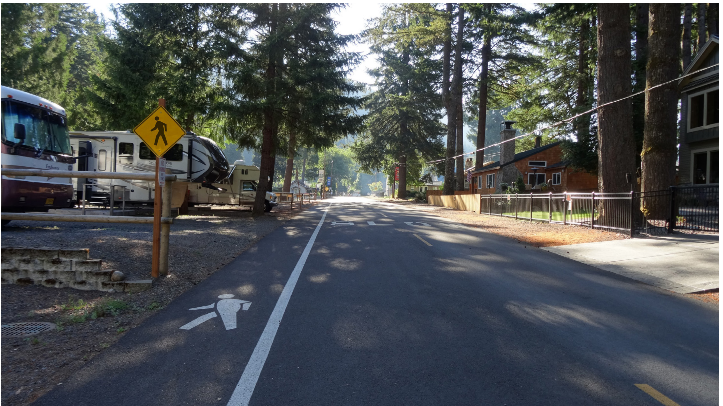
SE Maplewood Rd in Detroit, OR uses a pedestrian shoulder as an alternative to sidewalks.
