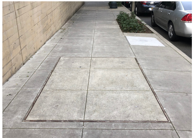
A concrete vault lid in the pedestrian through zone, matching the material of the surrounding sidewalk
