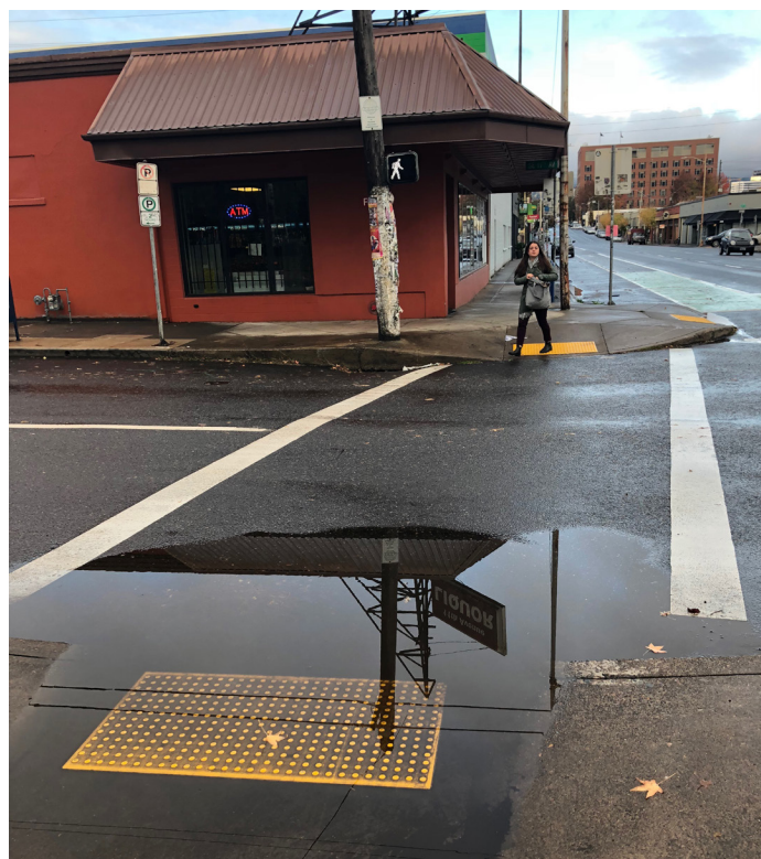
Pooling Water at Curb Ramp
