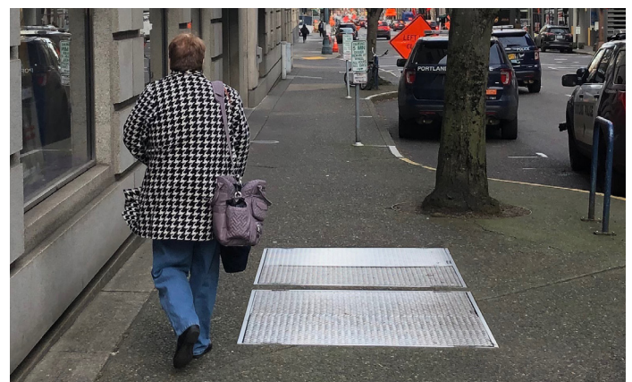
People walking tend to veer around metal vault lids in the sidewalk even when they are treated with “slip resistant” coating, effectively narrowing sidewalk capacity and obstructing the pedestrian through zone.
