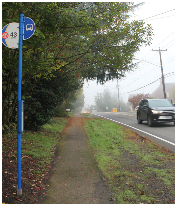
SW Taylors Ferry Rd in Southwest Portland. This historic example doesn't meet minimum widths, but provides an unpaved separation from the roadway.
