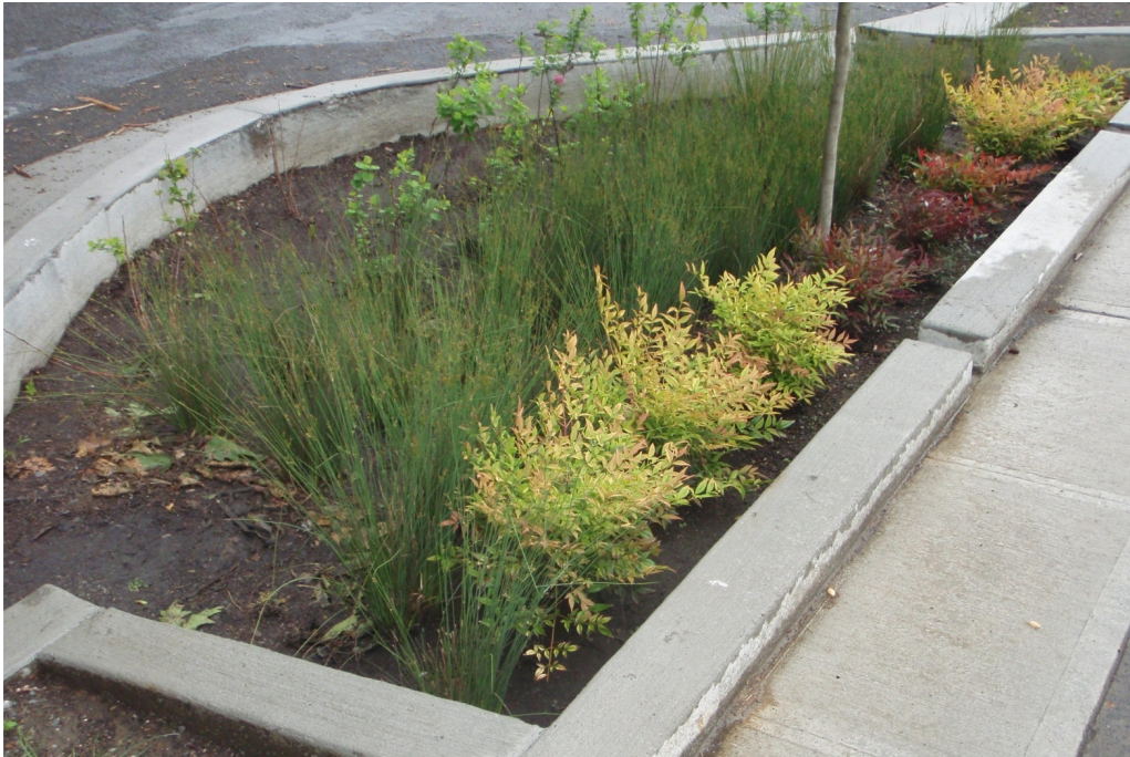
Bioswales filter water through native plants into the City's stormwater system, and introduce landscape elements to the right-of-way.
