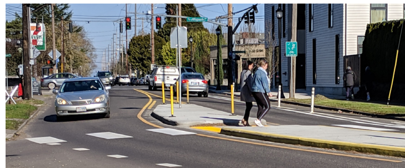
Median diverters at arterial / non-arterial intersections reduce the number of conflicts with turning vehicles that pedestrians must contend with and provide a central refuge to make crossings safer and more comfortable.
