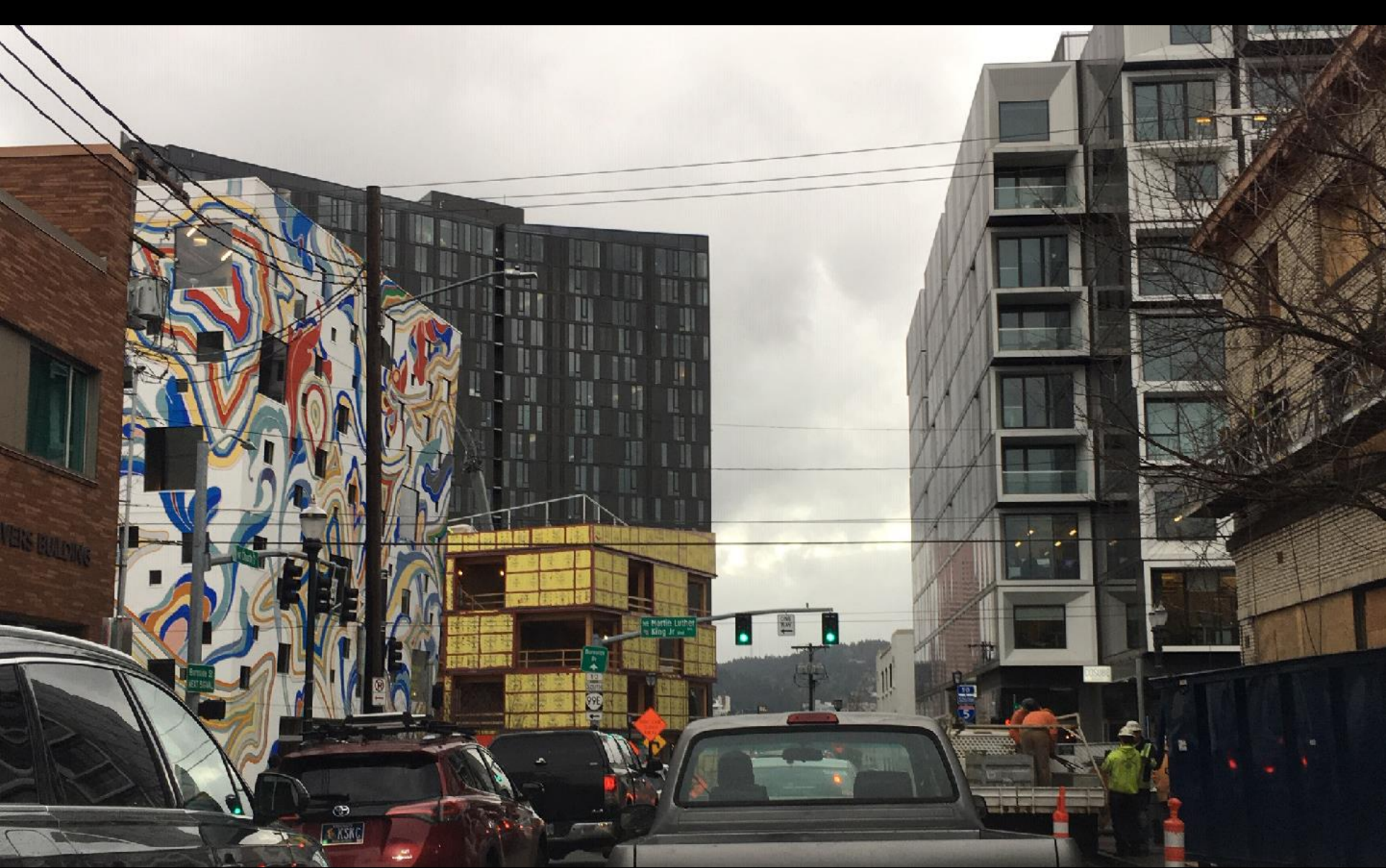
New Burnside Bridgehead buildings relate to nothing around them...not even themselves. Anything goes!
