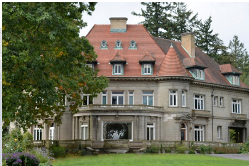
Pittock Mansion is a URM and vulnerable to earthquakes
