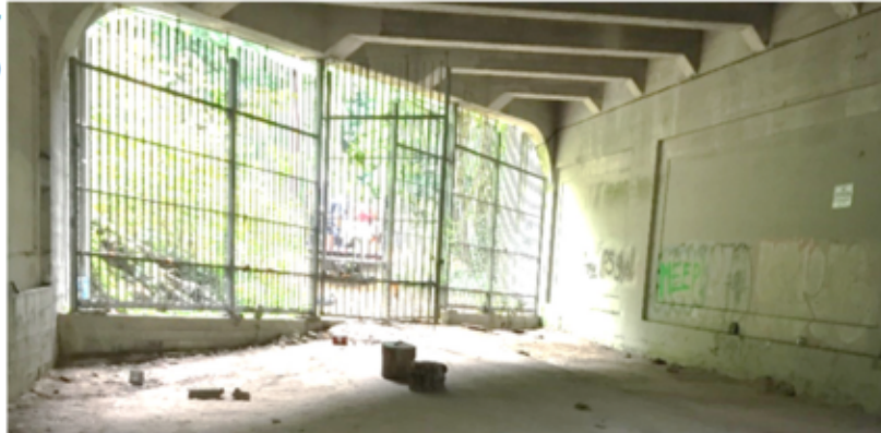
Underneath SW Jefferson St off-ramp, August 31, 2018
