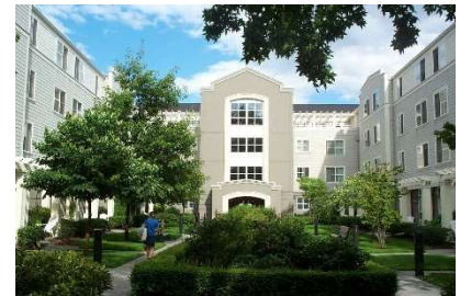
Examples of private and shared outdoor areas included in development typical of the RH zone.
